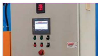
PLC Operated Electric Control Panel
